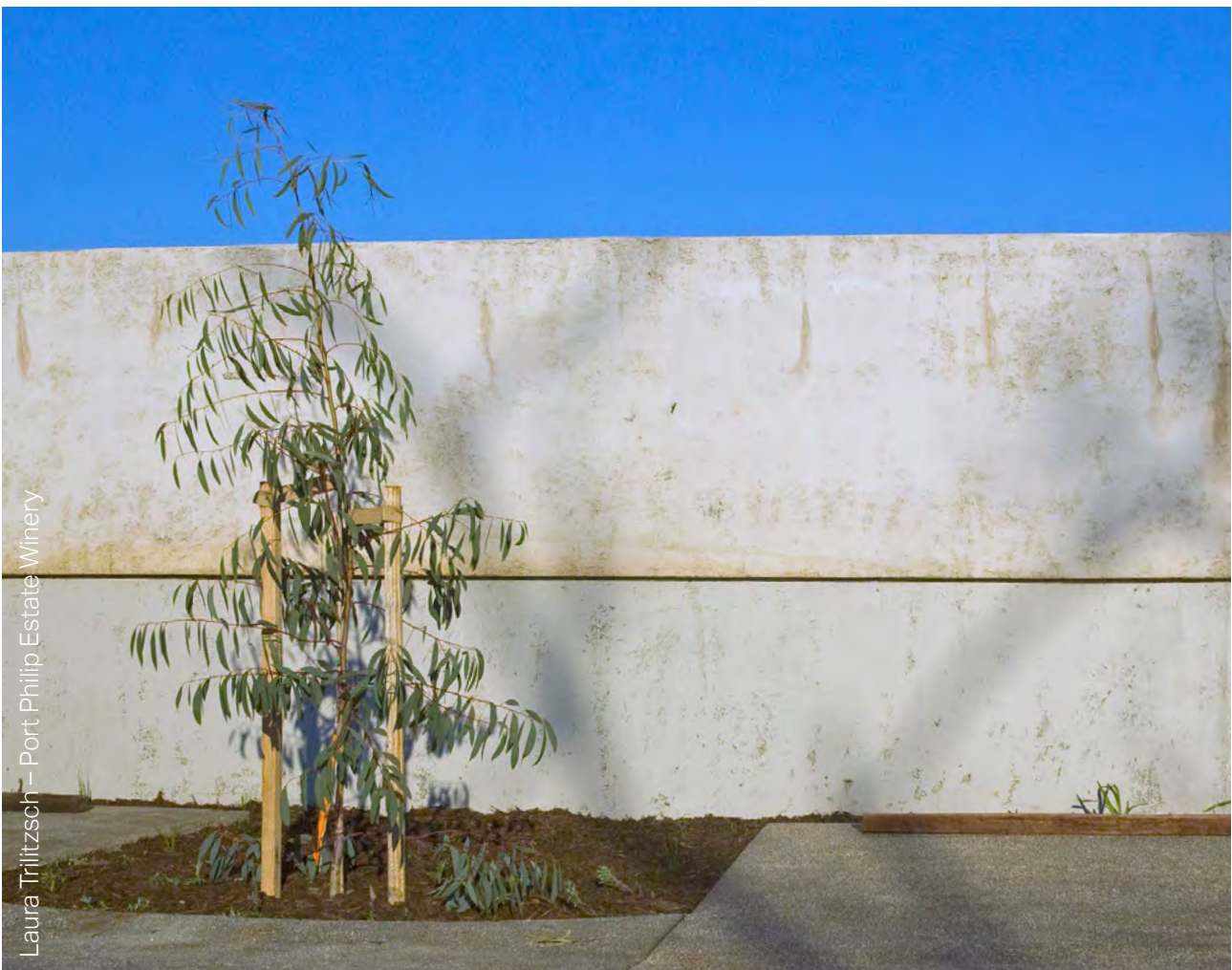
Figure 55: Example of rammed earth wall
