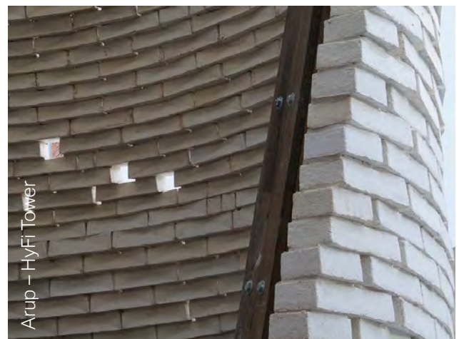
Figure 94: Example of mycelium building blocks
