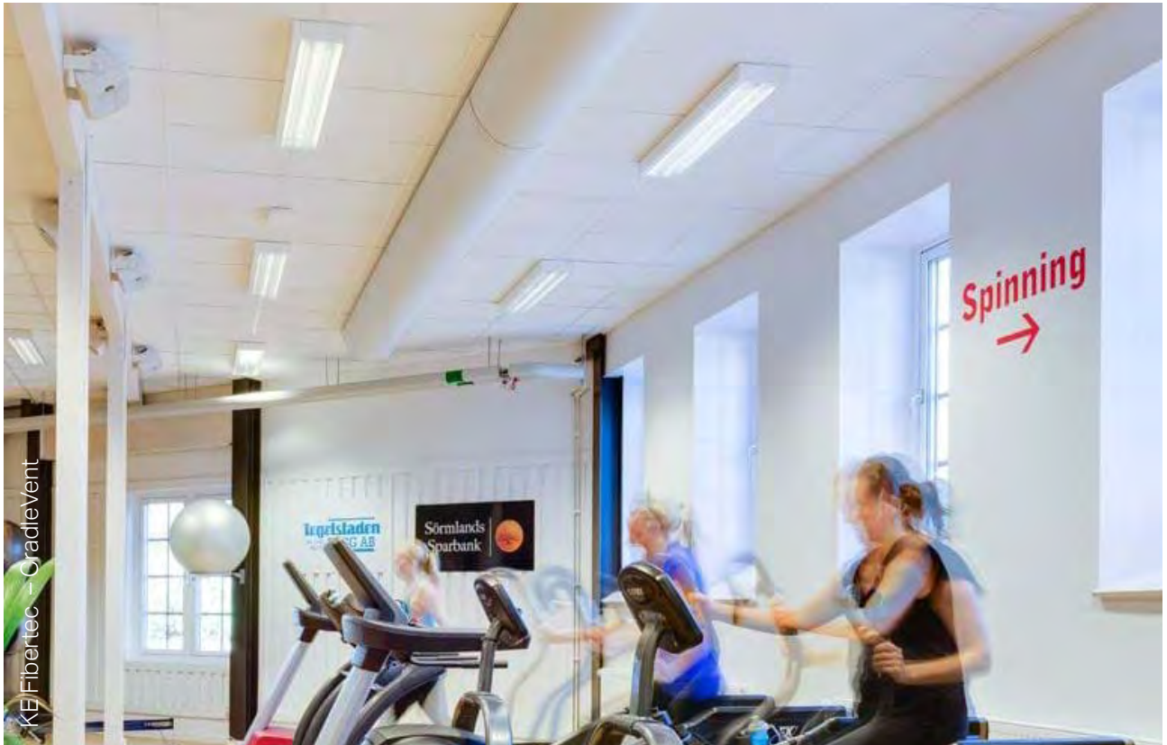
Figure 103: Example of cradle-to-cradle certified textile ductwork, Cradle Vent, used in a health center
