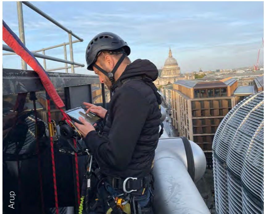
Figure 71: Façade inspection and maintenance considered from the outset
