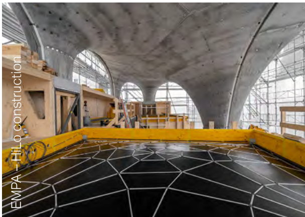
Figure 57: EMPA-ETH Zurich HiLo vaulted flooring system
