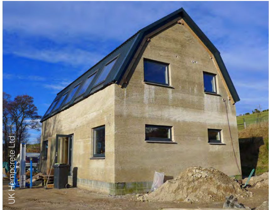
Figure 54: Example of hempcrete house
