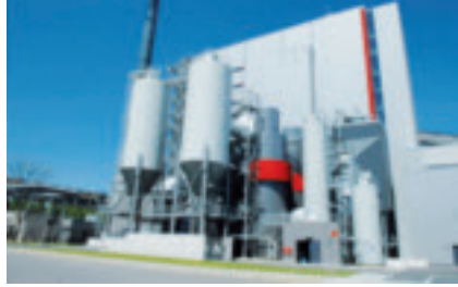
In 2010, Stora Enso commissioned a new 140 million Euro multifuel boiler at its Langerbrugge pulp and paper mill in Belgium. With an annual input capacity of 250000 – 300000 ton biomass and Refuse Derived Fuel, it generates 125MWh of power. Photo: Stora Enso
