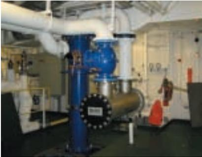
OptiMarin's OPTIMAR Ballast treatment System – based on solid separation and ultra violet irradiation – installed aboard the Regal Princess
