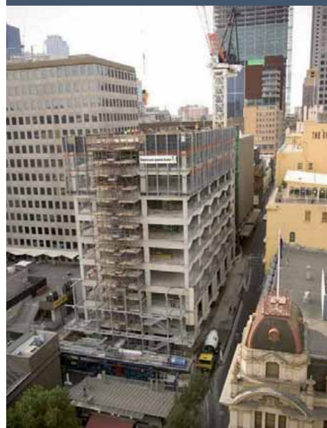
Example: Council House 2 in Melbourne, Australia with 6 Green Stars. The concrete used in the structure contains recycled concrete aggregate.
