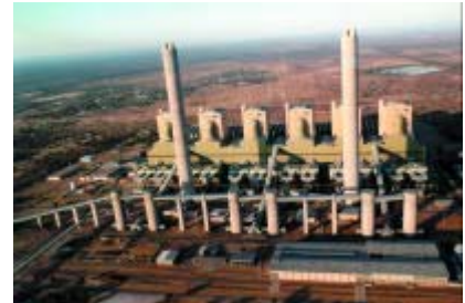
Matimba, one of Eskom's dry cooled powerstations
