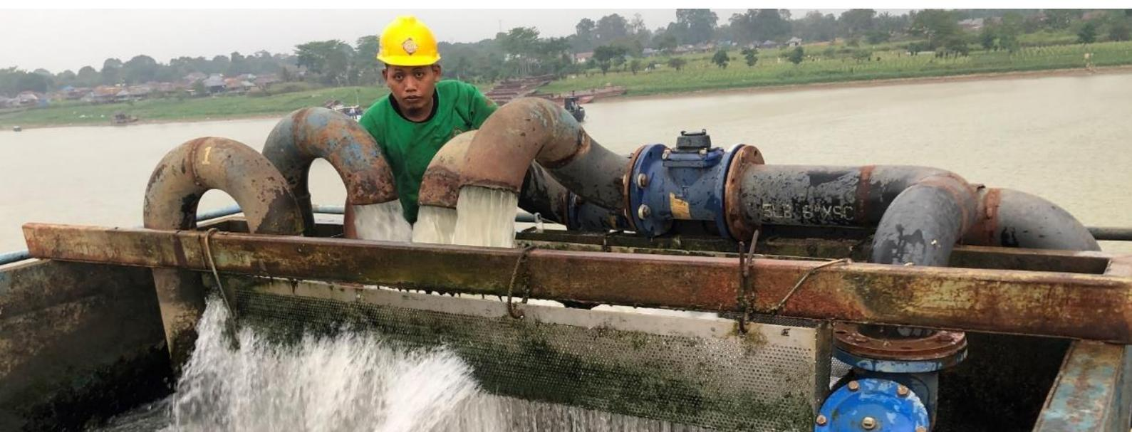
Picture 3: Water intake system with the water source, the river Batanghari in the background (image credits: Witteveen+Bos)
